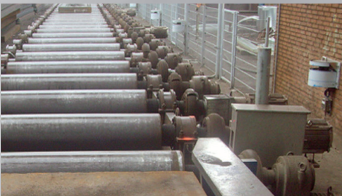
Slab tracking at the roller table
